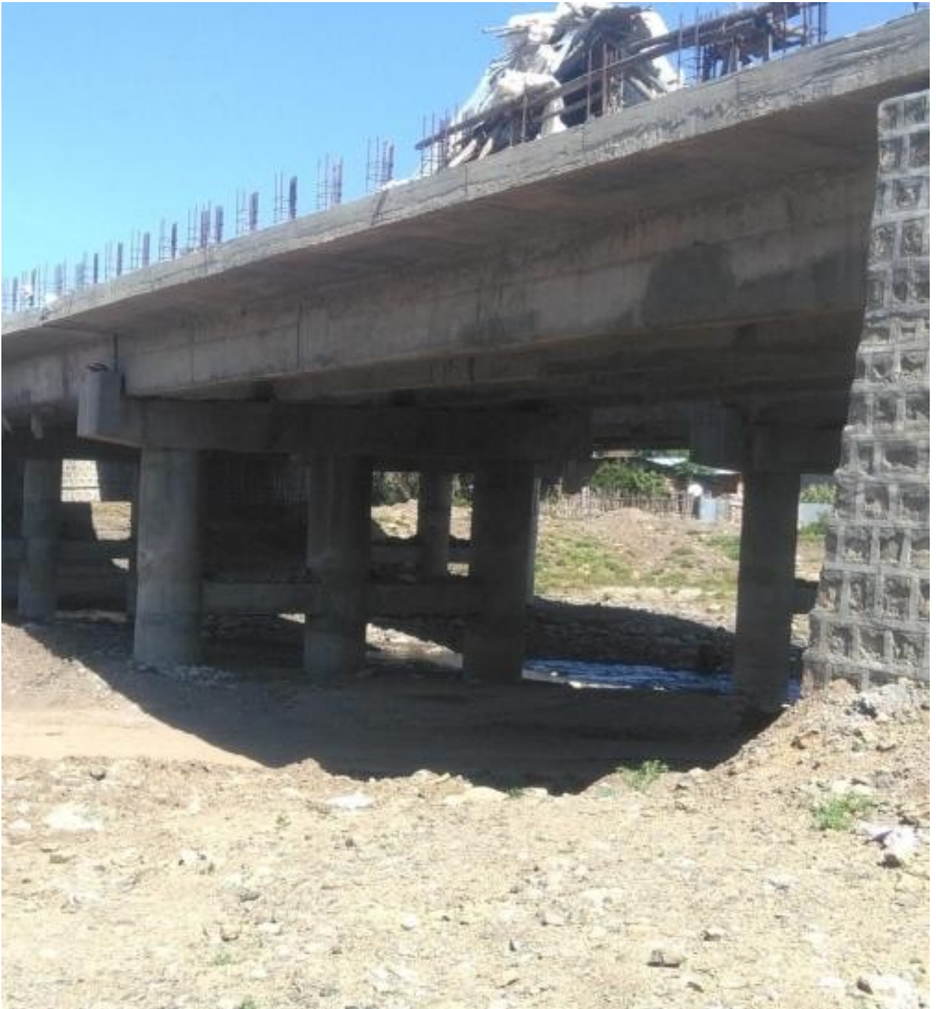
Bridge @0+100(60m span)
