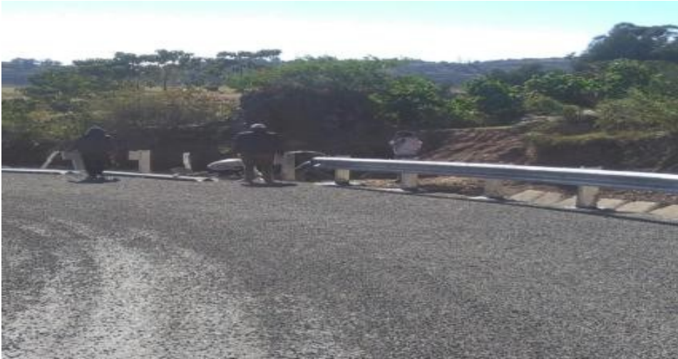
Guard rail installation work
