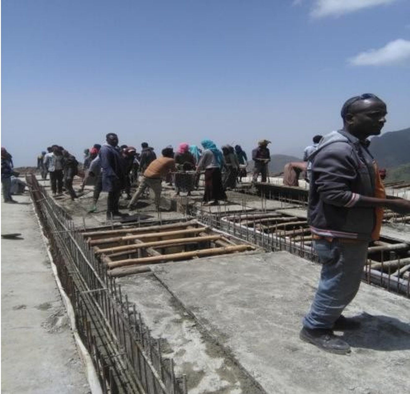
Shimelis over pass bridge girder concrete casting
