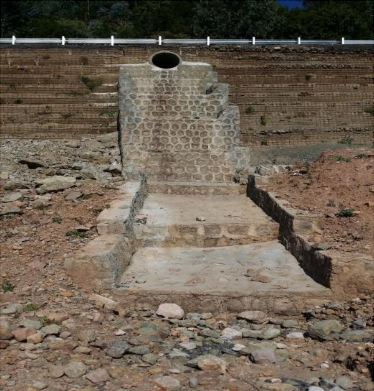
Reinforced earth wall with pipe @km29+100
