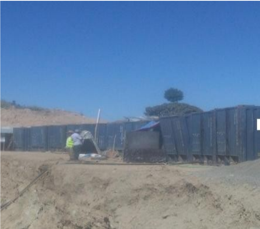
Bitumen boiling activity
