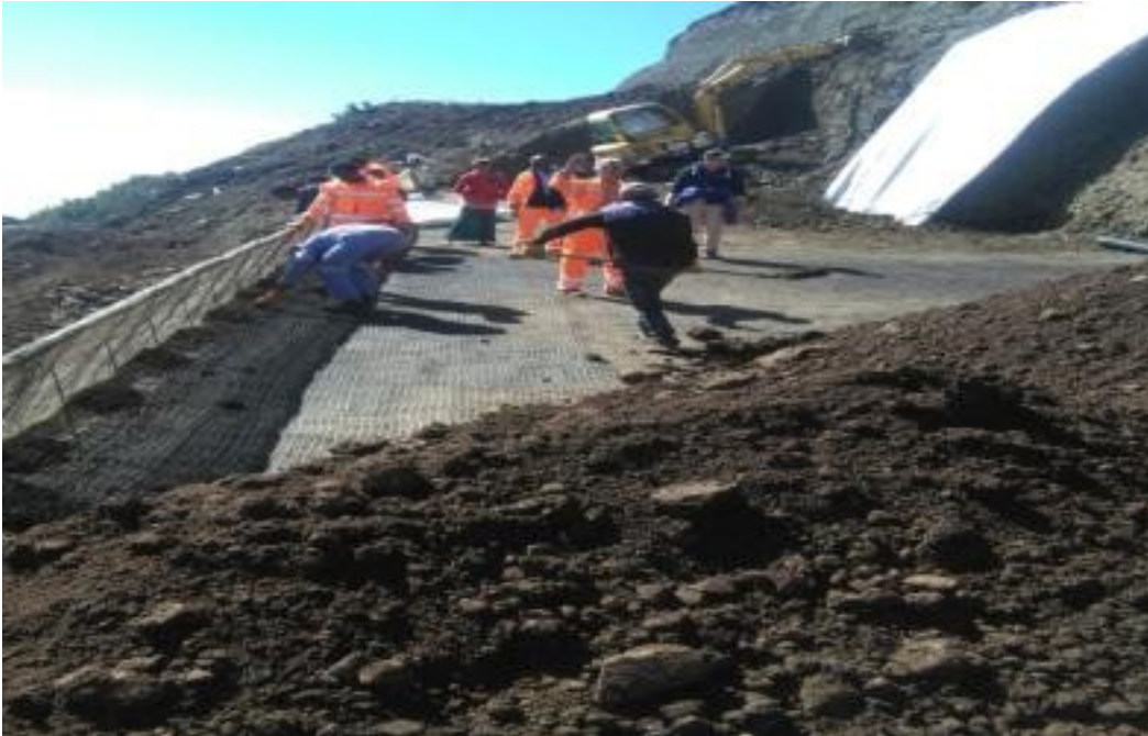
Mechanical stabilized earth wall work
