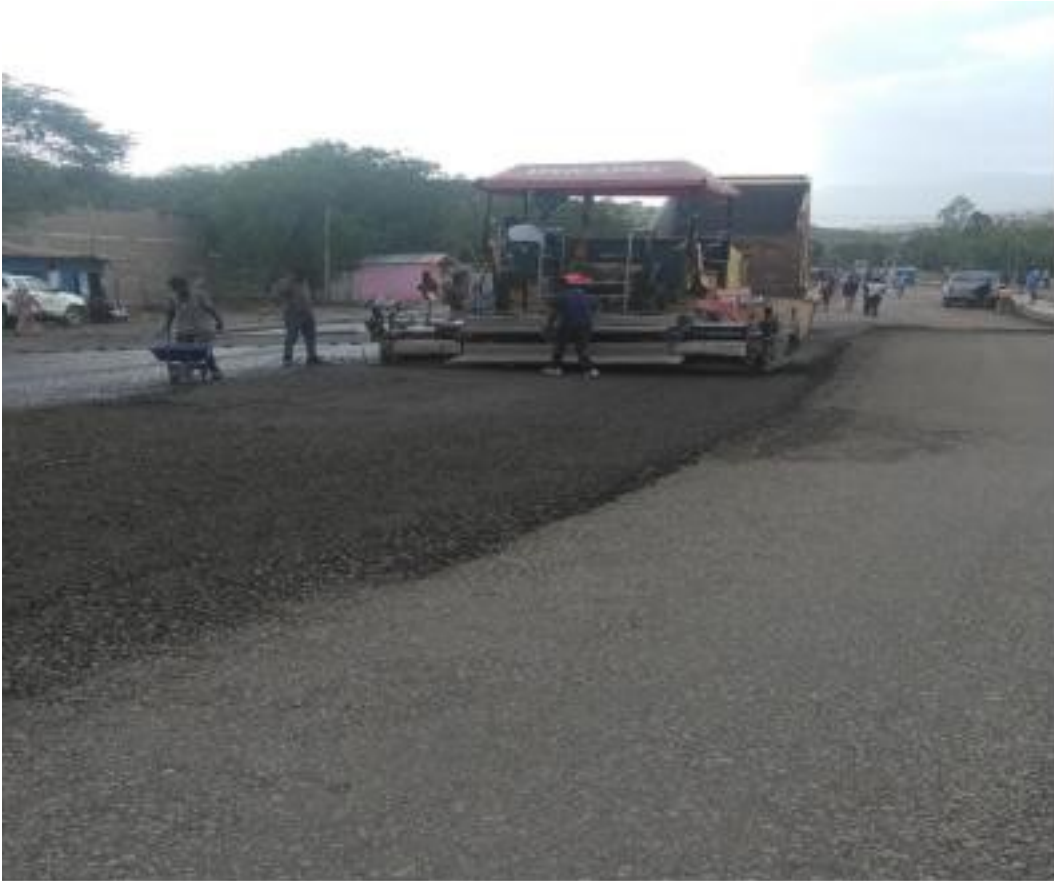
Base course placing
