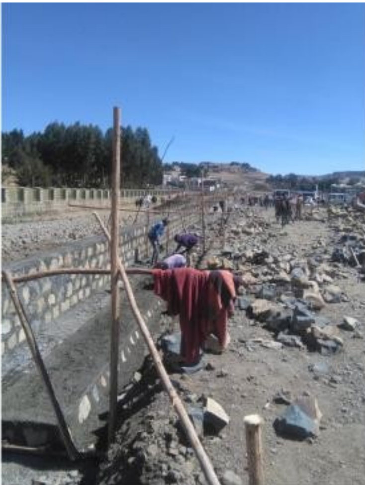
Town ditch masonry work
