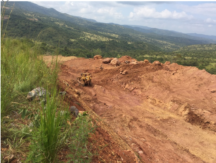
@km 84+500 common excavation
