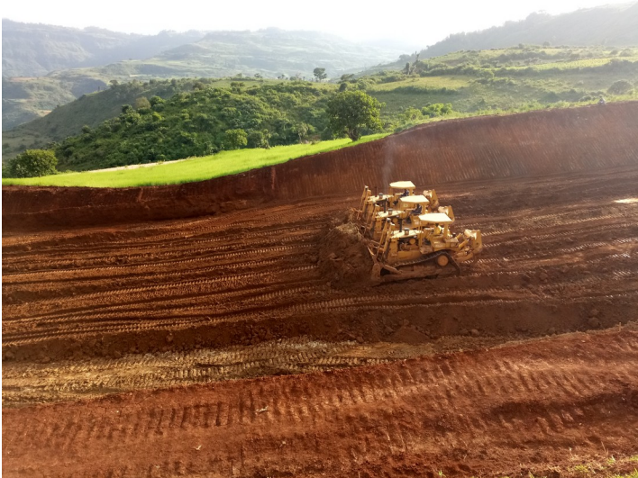
@km 68+800 Common Excavation
