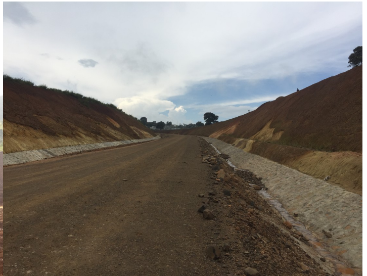
Around 93+700 Trapezoidal Ditch Construction
