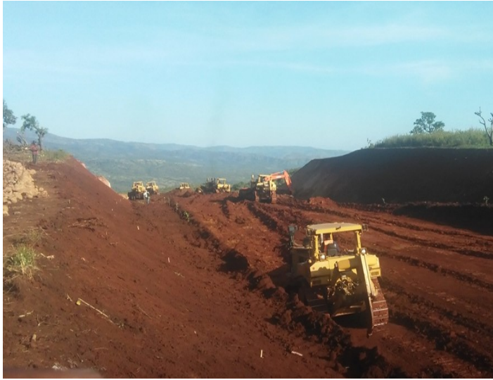
@km 72+230 common excavation
