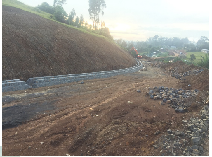
800 Masonary Town Ditch Construction
