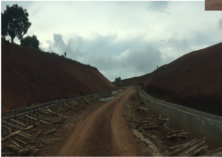
Around 89+600 Concrete UDitch Constructio
