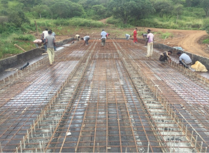
@82+089 Reinforcement Bar Placing
